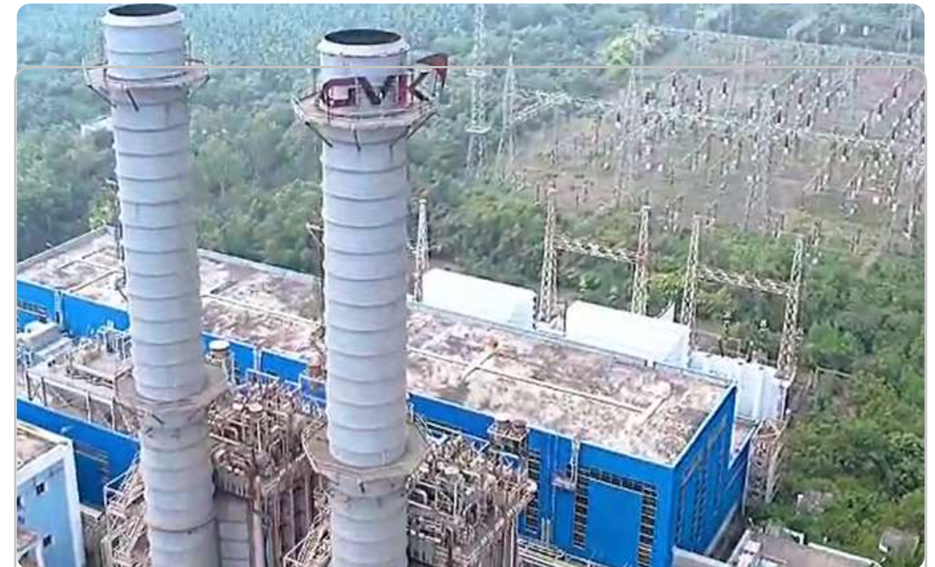
Drone View of the Plant
