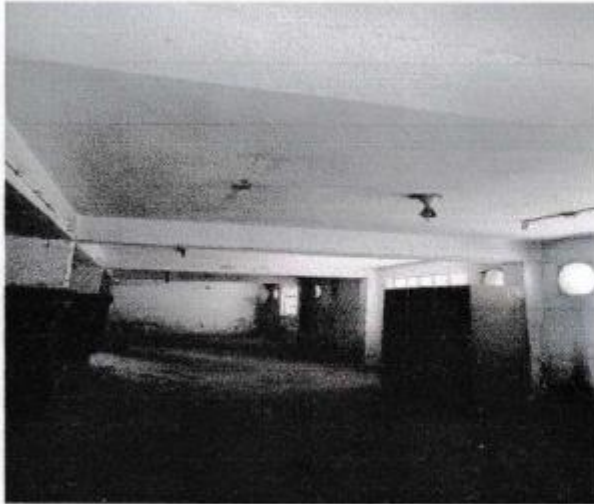
GF Area Covered with RCC Slab
